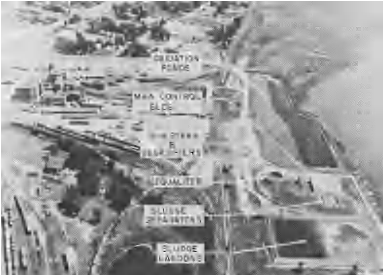
Figure 2. Full scale anaerobic contact waste treatment plant, Wilson & Co. Inc., Albert Lea, Minnesota USA
