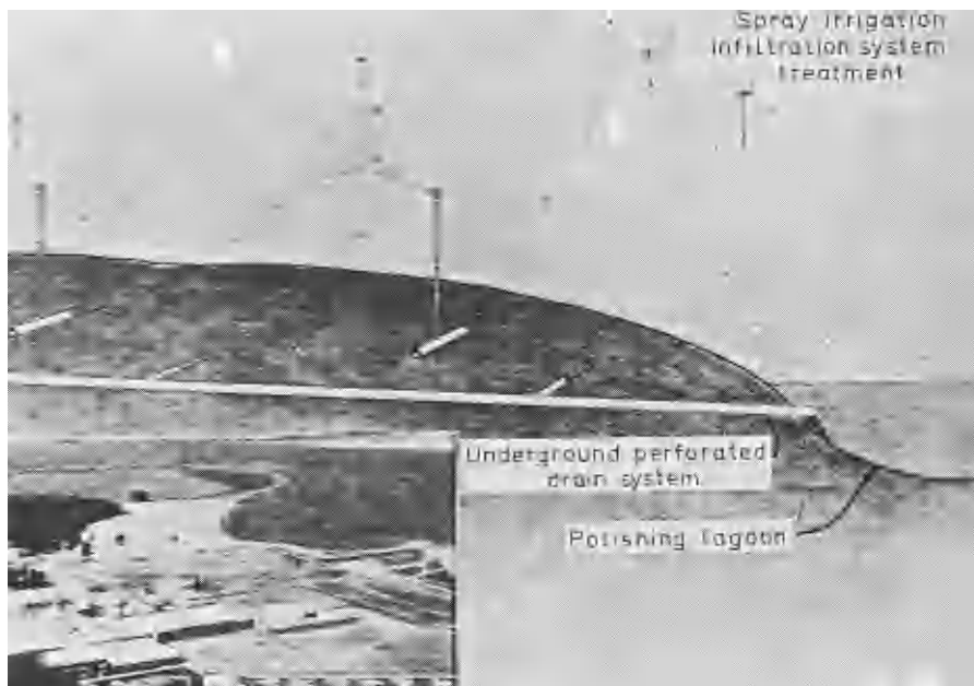
Figure 13. Spray irrigation infiltration system treatment.
