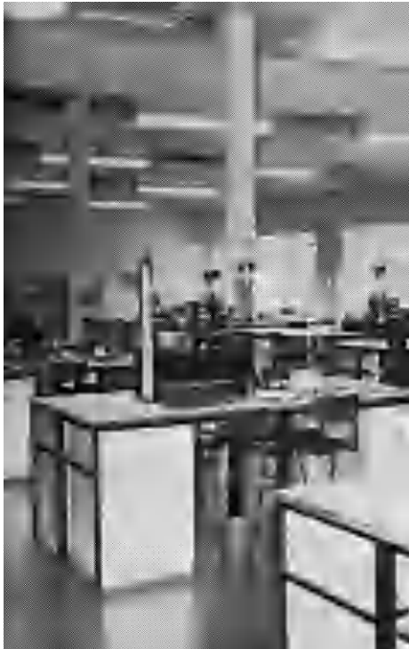
Figure 3. Electricity is provided by units suspended from the ceiling which are readily removed when not required. PAC—facing page 108
